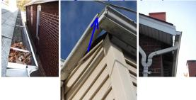
8. Minor Repair Downspouts: Aluminum. Be sure to keep the splash pads properly positioned to help prevent erosion and to direct water out and away from the foundation and sidewalks.
