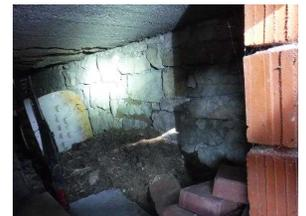
11. Marginal Ventilation: Absent - - All unconditioned crawl spaces should be provided with flow-through ventilation with side vents to the exterior. The existing panels could be removed and replaced with a new frame and screen sized for the opening or vents could be cut into the existing panels to allow air to flow through the crawl space. The screen should be a minimum 1/8x1/8" metal hardware mesh to help prevent the entry of insects and rodents.
