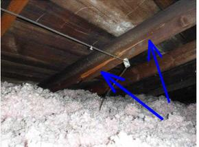
8. Acceptable Trusses: Manufactured trusses at REAR ADDITION - - No damage requiring repair was visible. However, stains are present on the wood members from leakage through the roof.
