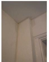
3. Minor Repair Walls: Drywall. Plaster. - Some common plaster cracks and patched areas are present. This is common to observe in a house of this age. A painting contractor could easily repair these areas and paint to match.
